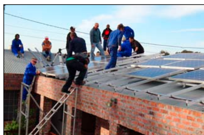
Installateurtraining 2012 in Kapstadt
